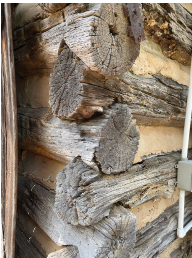
V - notching above is considered to be exclusive Cherokee period construction method.
