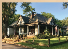
118 Park St Bishop-Bradley House (1905)
