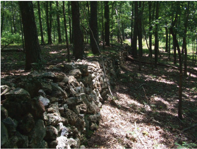
Example of dry stack wall construction running about 500 feet in length.
