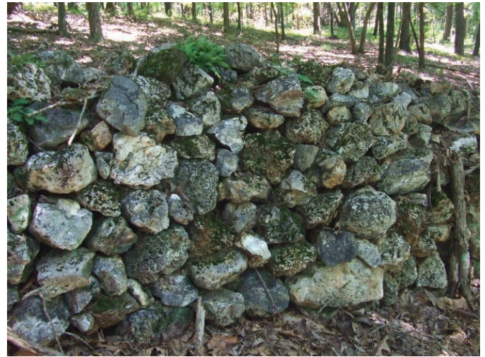
Example of dry stack wall construction running about 500 feet in length.
