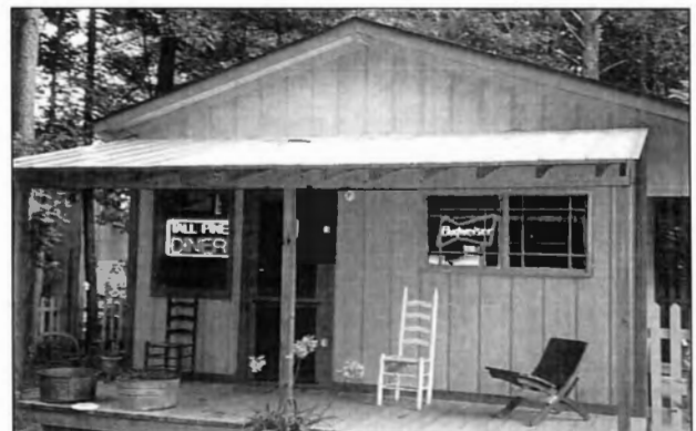
The Tall Pine diner is one of four buildings in the 1930s village being constructed by Jane and James McElreath on their property on Old Alabama Road.
