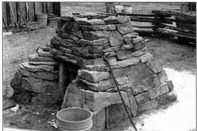
Miniature iron furnace, built by the Red Top Park staff, produced iron from ore collected along the banks of Lake Allatoona.
