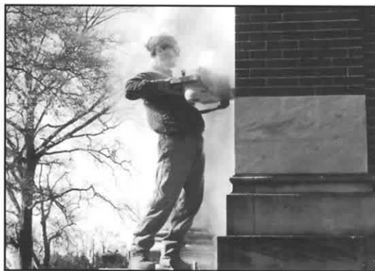
Scott Swanson uses a masonry saw to cut into the mortar between bricks lying just above the cornerstone.
