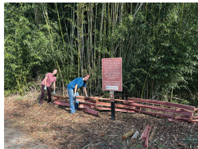
Split-railers are work!
