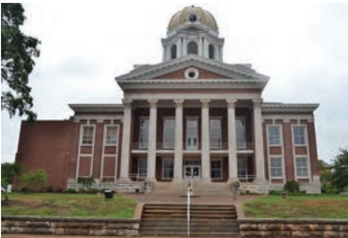
2023 Courthouse view (note extension on left side)
